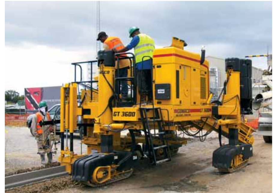
A GT-3600 slipforms curb at a new power plant in Trinidad.
