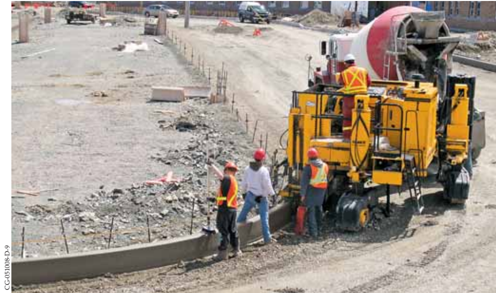
This GT-3600 slipforms a 16 inch (406 mm) curb in Canada.
