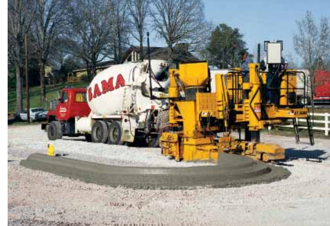
A GOMACO GT-3600 slipformed a curb and gutter radius string-free using 3D controls for the first time in March 1999.
