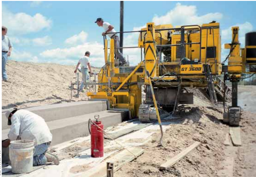
A project for 10 rows of stair-stepped risers within a new football stadium is completed in five passes around the facility with the GT-3600.
