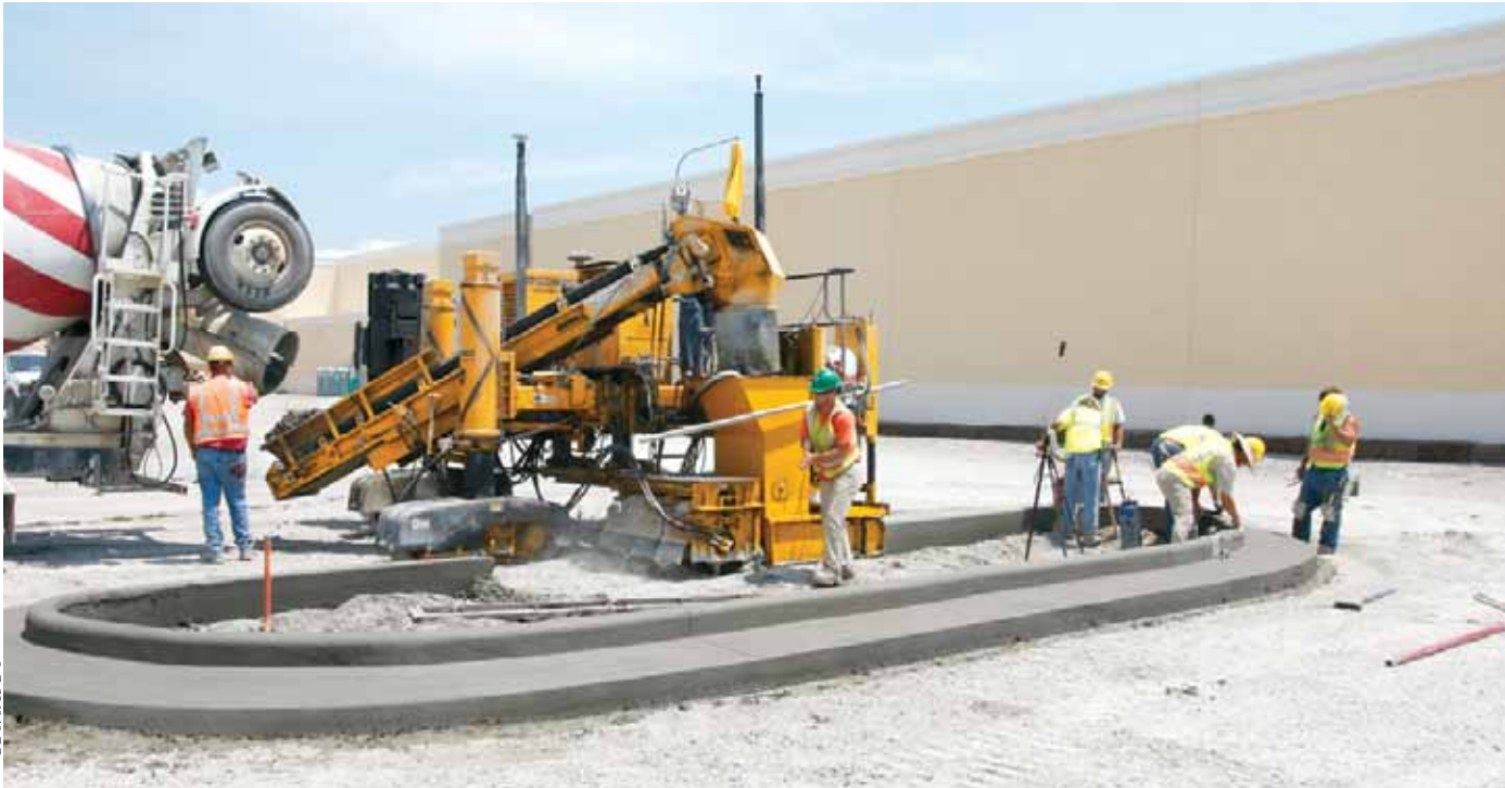
The GT-3600 slipforms the tight radii of parking lot islands with ease after having loaded the hopper and charging conveyor prior to starting the island.
