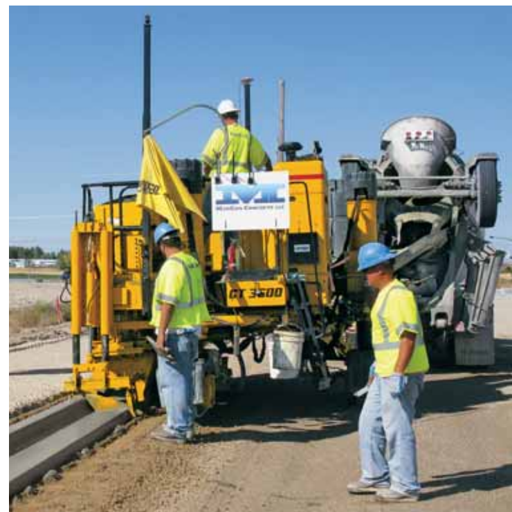
Stringless curb and gutter is slipformed on a new parking lot project with 3D stringless controls.
