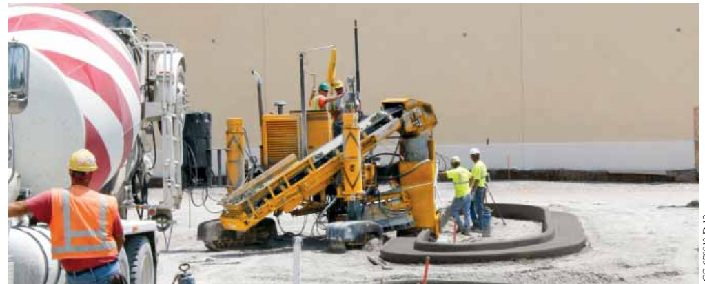
A GT-3600 with 3D stringless controls slipforms the tight radii of parking lot islands.
