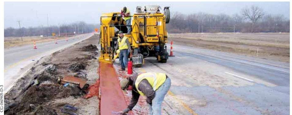
A GT-3600 with a custom-built mold slipforms a 24 inch (610 mm) median strip at a 30 degree angle with red dyed concrete.
