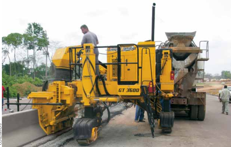
A GT-3600 slipforms a safety barrier in Equatorial Guinea.
