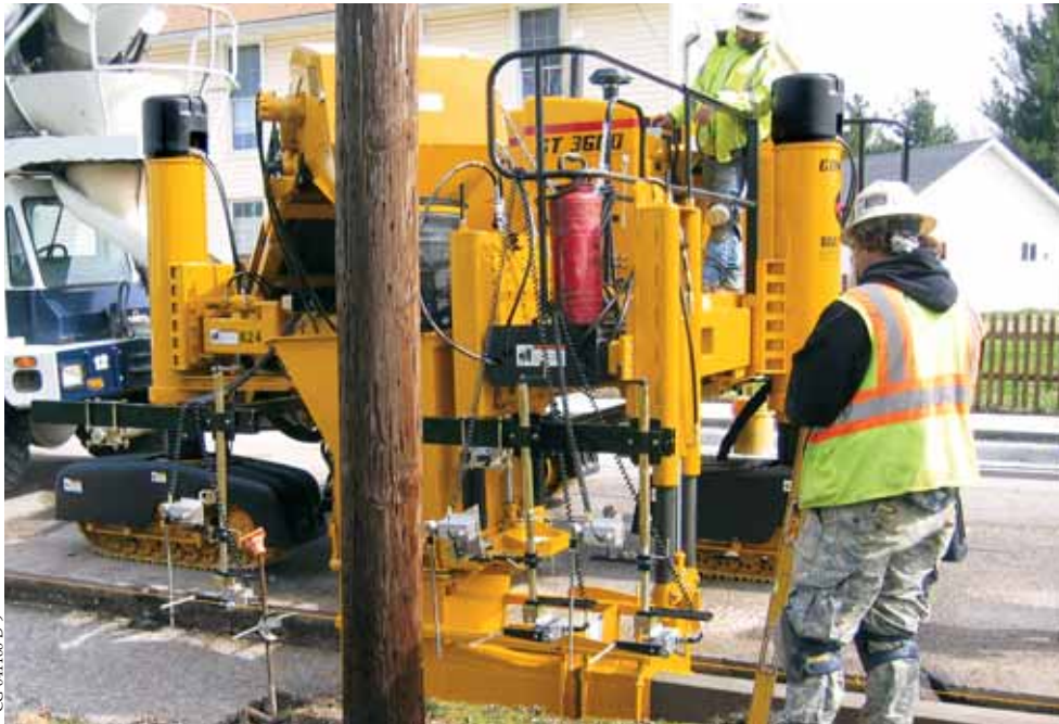
The operator uses the sideshifting capabilities to achieve minimum-clearance as the GT-3600 passes by a utility pole on a rehabilitation project.
